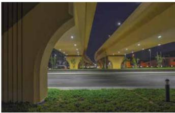
• Cast in Situ Deck Slap (Box Section)
