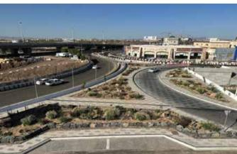
• Distance: 900 LM in two directions with three traffic lanes in addition to a path for buses movement in each direction.
